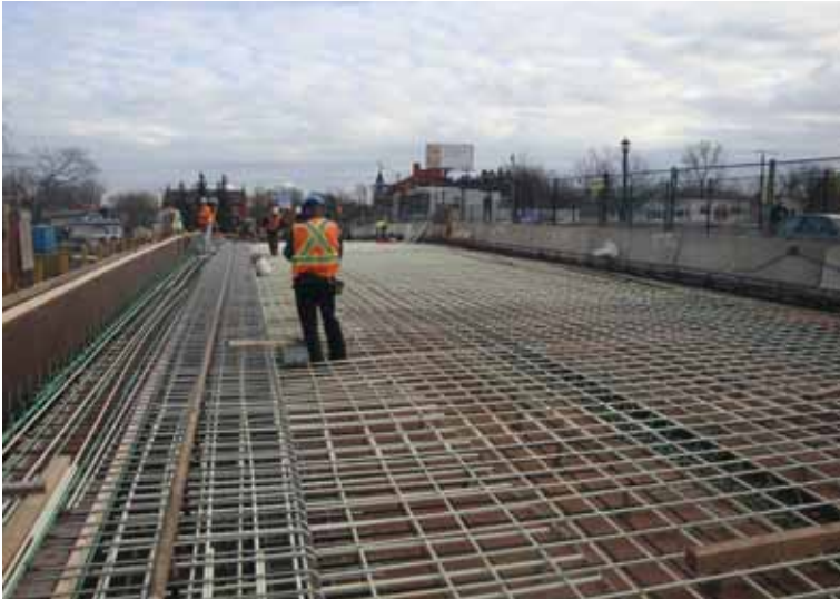
Weightman Bridge, Niagara Falls, Ontario, Canada
