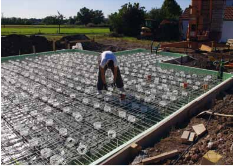
Floor slab in Dr. Moldan's residence in Iphofen
